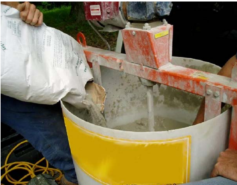
FIGURE 15-30: ANOTHER GROUT MIXING MACHINE
