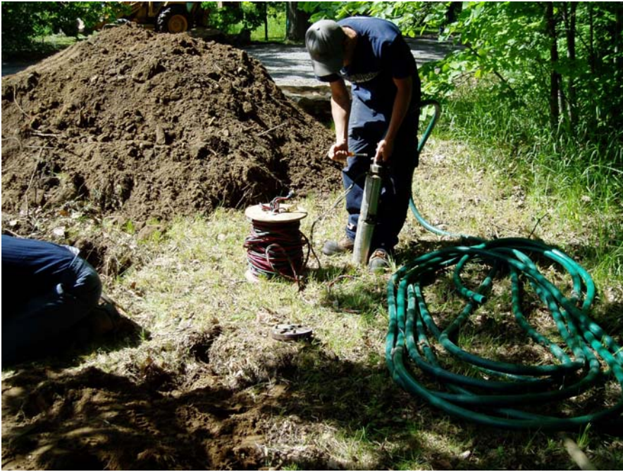
FIGURE 15-27: PREPARING TO INSTALL SUBMERSIBLE PUMP
