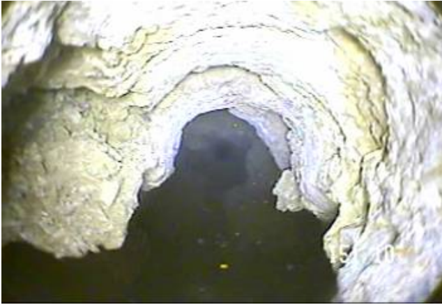
FIGURE 15-6: VIDEO TECHNOLOGY USED WITHIN A DRILLED WELL
