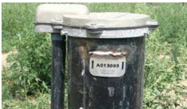
FIGURE 15-10: WELL TAG ON DRILLED WELL
