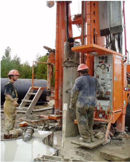
FIGURE 15-15: REMOVAL OF WELL CASING
