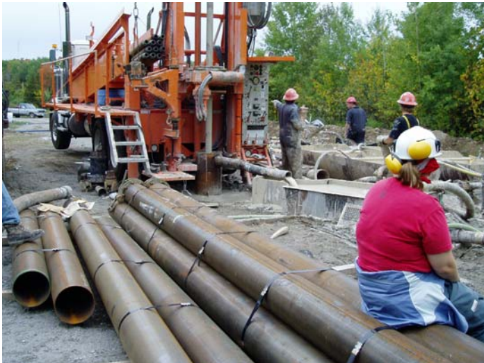
FIGURE 15-41: FLOWING WELL AT BACK OF DRILLING RIG
