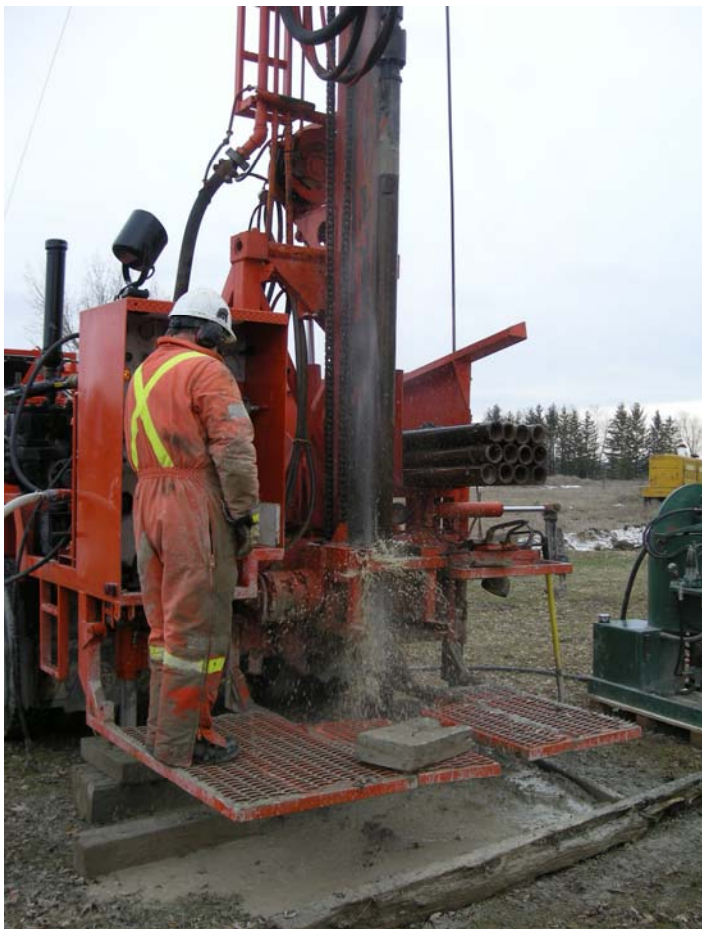
FIGURE 15-28: COMPRESSED AIR REMOVAL OF DEBRIS
