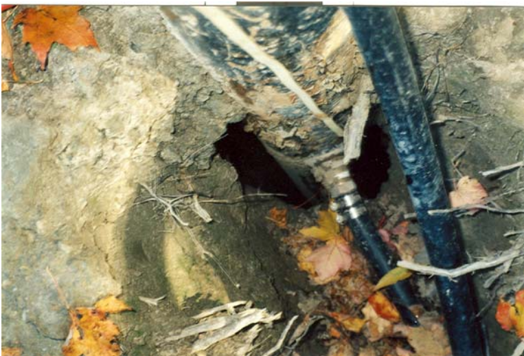
FIGURE 15-23: EXTERIOR OF PITLESS ADAPTER
