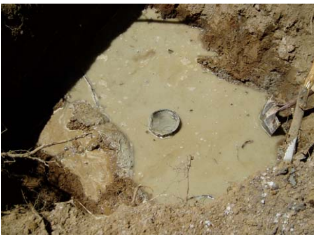
FIGURE 15-36: CUT CASING WITH ABANDONMENT BARRIER
