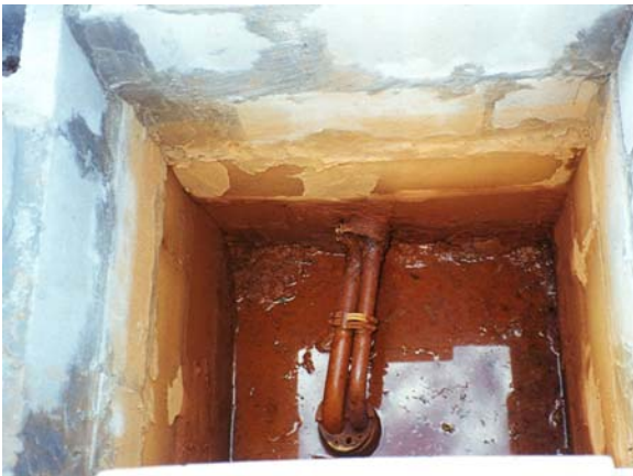
FIGURE 15-5: DRILLED WELL IN A WELL PIT
