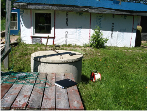
FIGURE 15-2: TYPICAL DUG WELL
