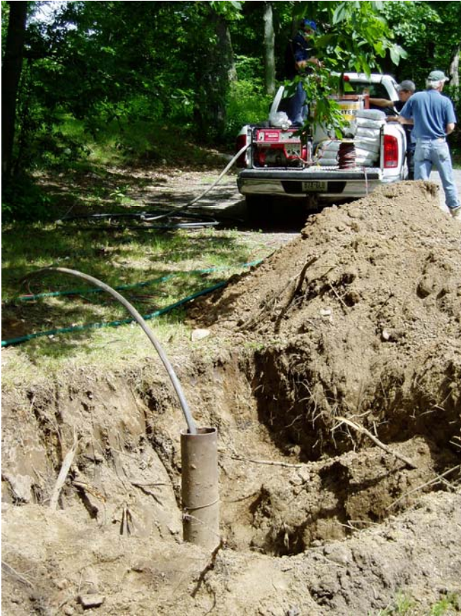
FIGURE 15-31: TREMIE PIPE INSTALLED INTO DRILLED WELL
