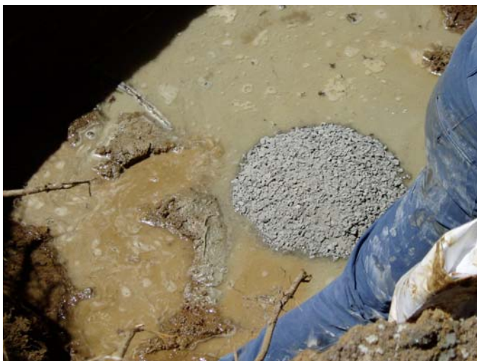
FIGURE 15-37: PLACING BENTONITE PELLETS ON TOP OF ABANDONMENT BARRIER
