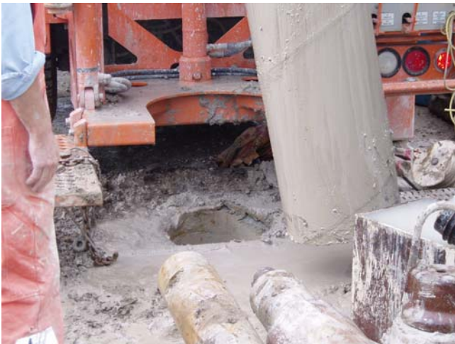
FIGURE 15-16: REMOVAL OF WELL CASING
