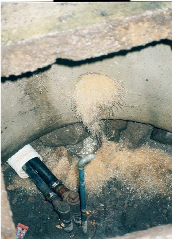
FIGURE 15-25: WATERLINES, AIR VENT AND SEAL TO BE REMOVED
