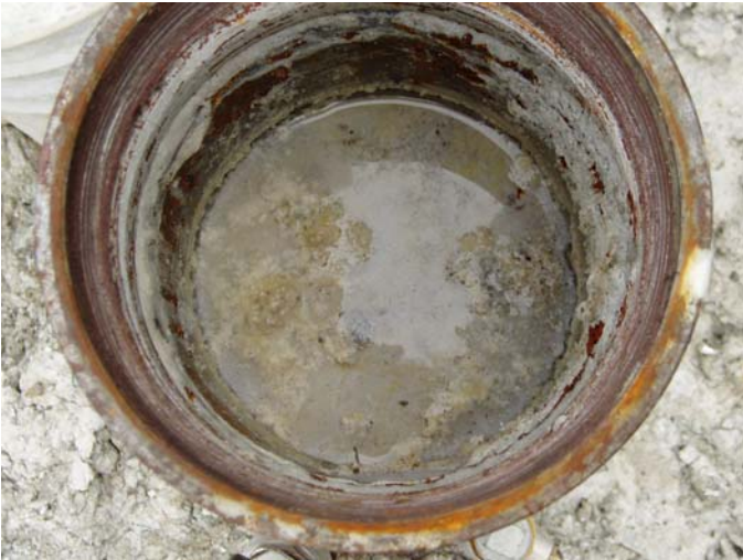
FIGURE 15-22: DRILLED WELL PARTIALLY FILLED WITH CONCRETE
