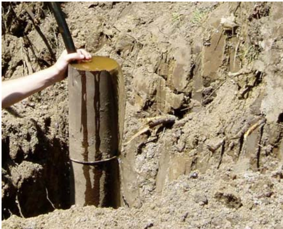
FIGURE 15-33: PLUGGING MATERIAL DISPLACING UNCONTAMINATED WATER
