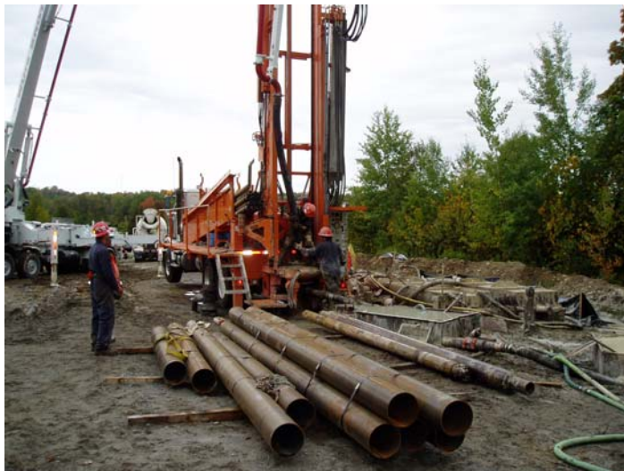
FIGURE 15-43: TREMIE PIPE GOING INTO FLOWING WELL
