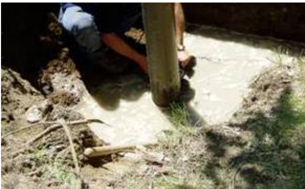
FIGURE 15-35: REMOVING 2 METRES OF WELL CASING
