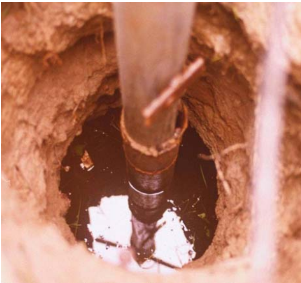
FIGURE 6-4: VISIBLE OPEN AND LARGE ANNULAR SPACE AROUND DRILLED WELL
