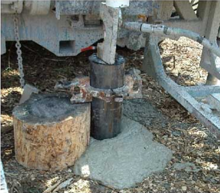
FIGURE 6-14: PUMPING GROUT DOWN TREMIE PIPE – INSIDE CASING
