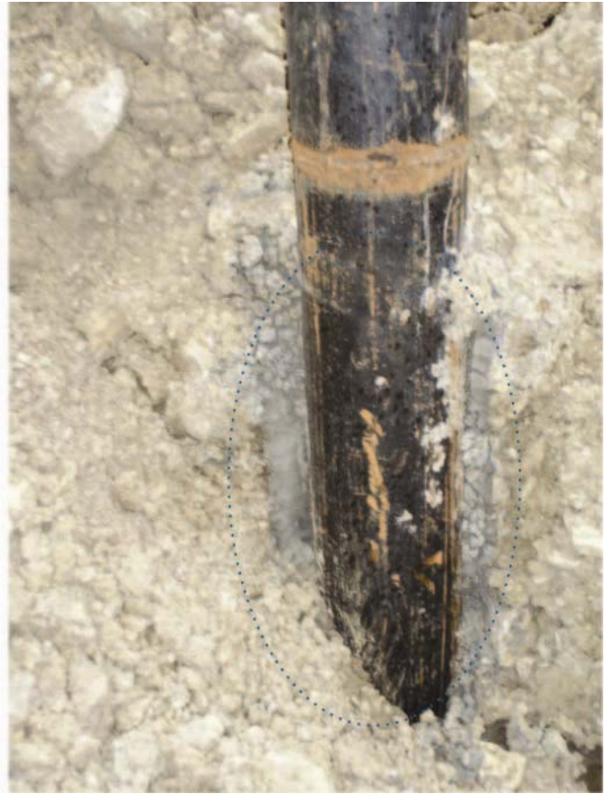
FIGURE 6-21: BENTONITE GROUT IN ANNULAR SPACE
