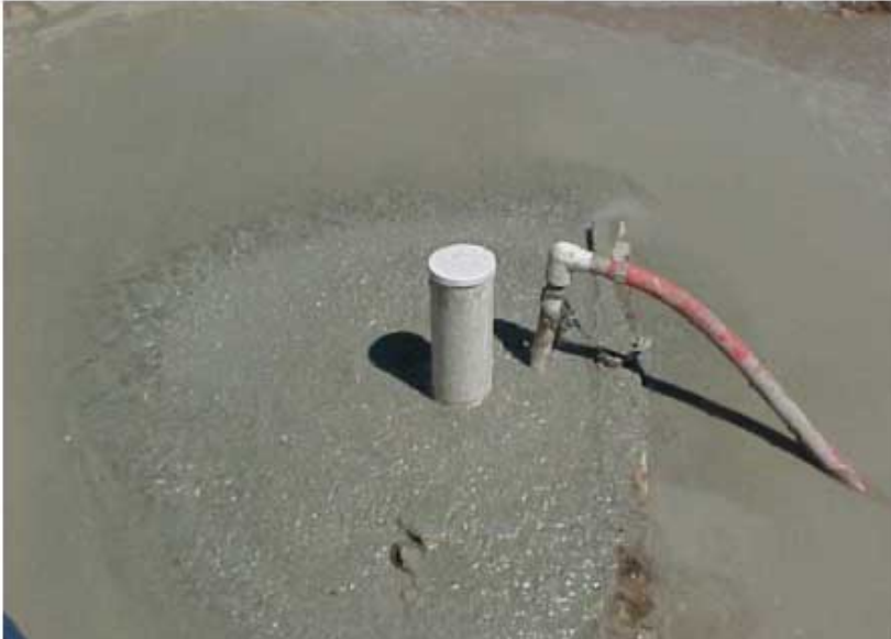
FIGURE 6-19: TREMIE REMAINS IN HOLE DURING GROUT PLACEMENT
