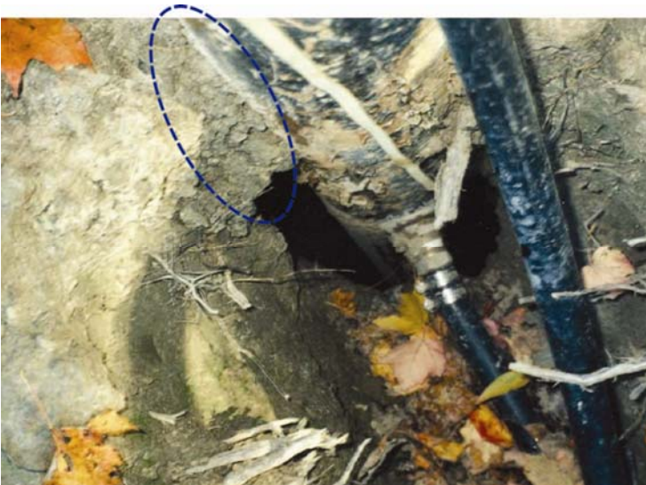
FIGURE 6-5: VISIBLE OPEN ANNULAR SPACE BELOW PITLESS ADAPTER AND HORIZONTAL WATERLINE TO THE BOTTOM OF THE CASING
