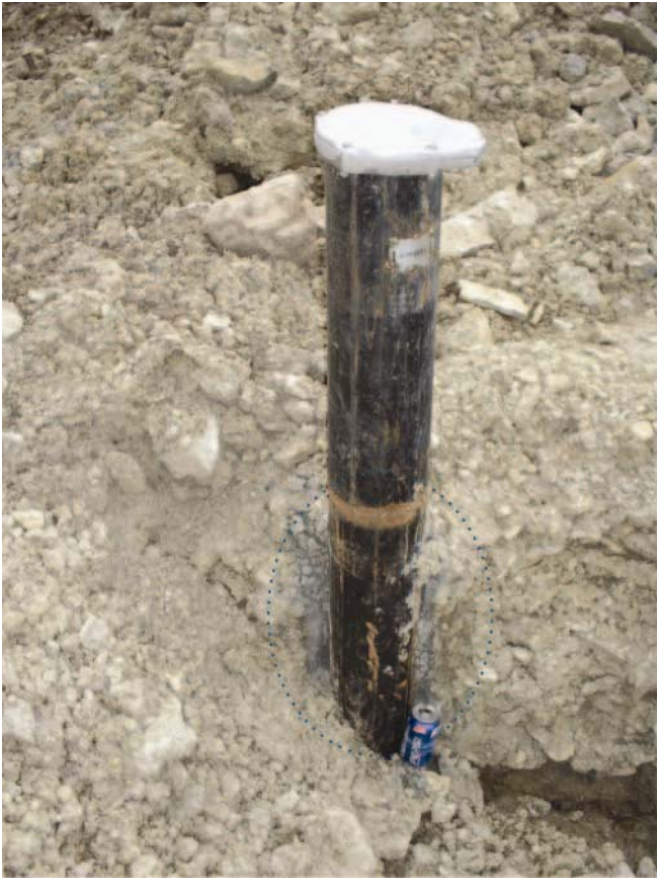
FIGURE 6-20: HOLE EXCAVATED BESIDE DRILLED WELL
