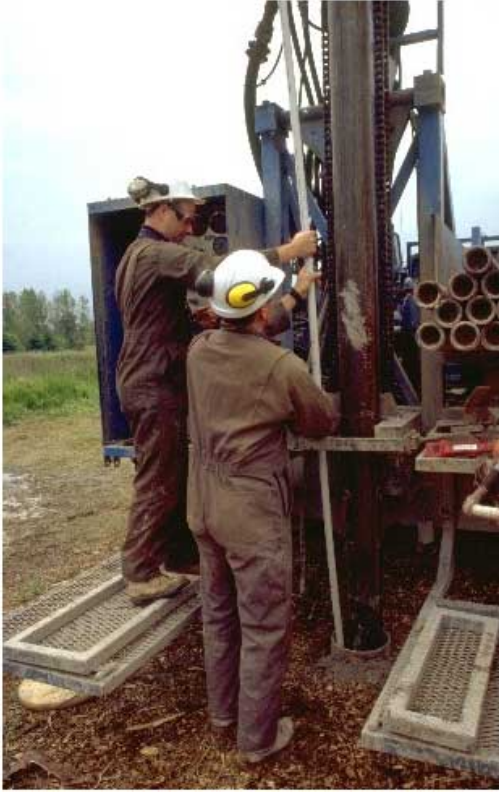
FIGURE 6-17: INSTALLING TREMIE PIPE OUTSIDE CASING
