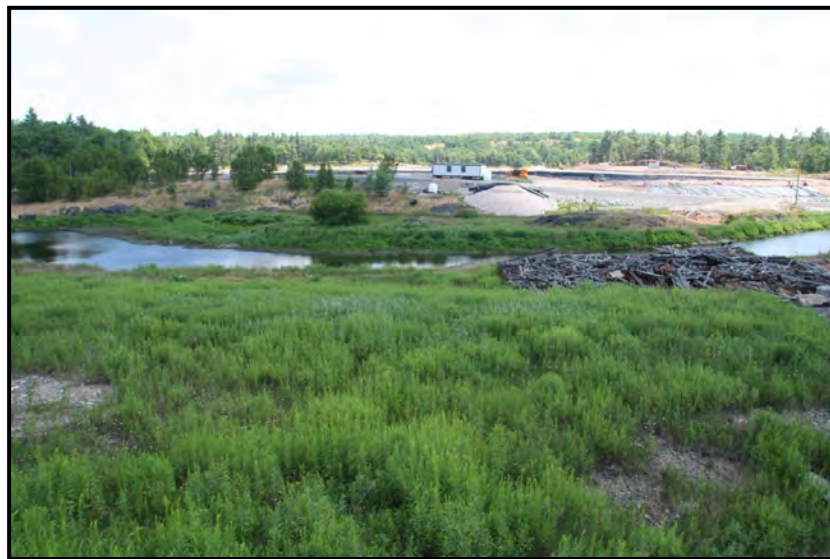
Plate 77: Looking across the Moira River to the Tailings Pond remediation, 2011.
