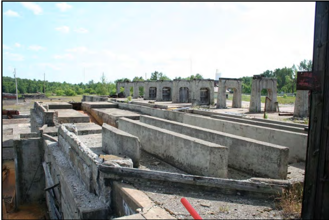
Plate 61: Supportive concrete slabs.
