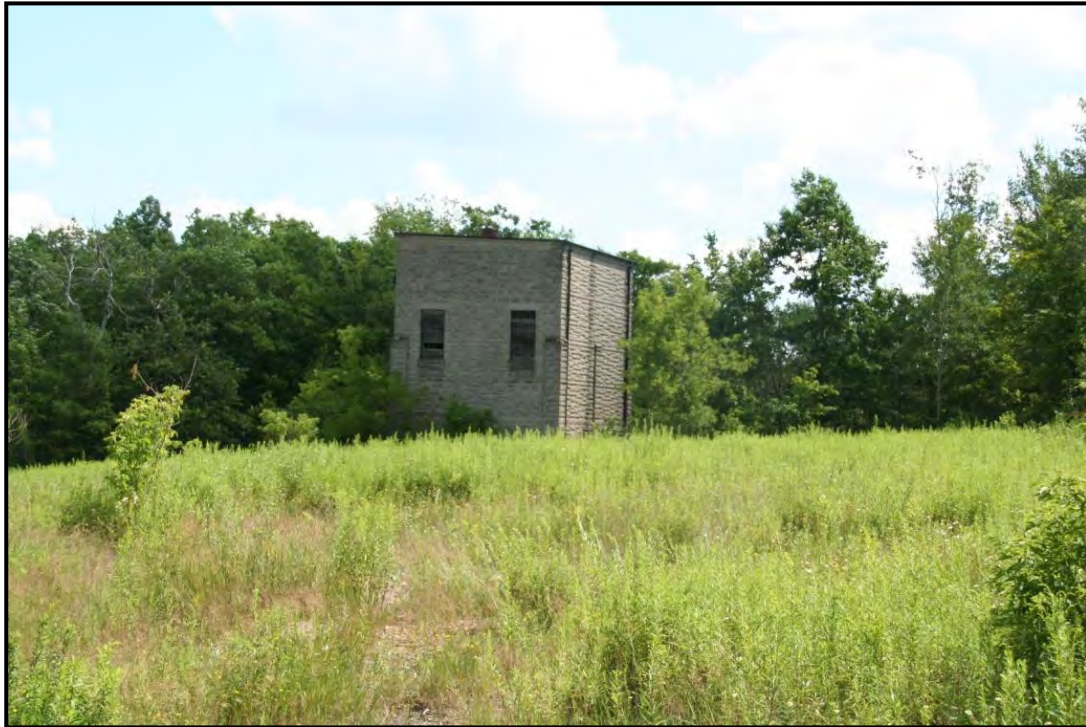
Plate 51: Transformer Building; grass field in foreground was location of powerhouse and Chemical Building.
