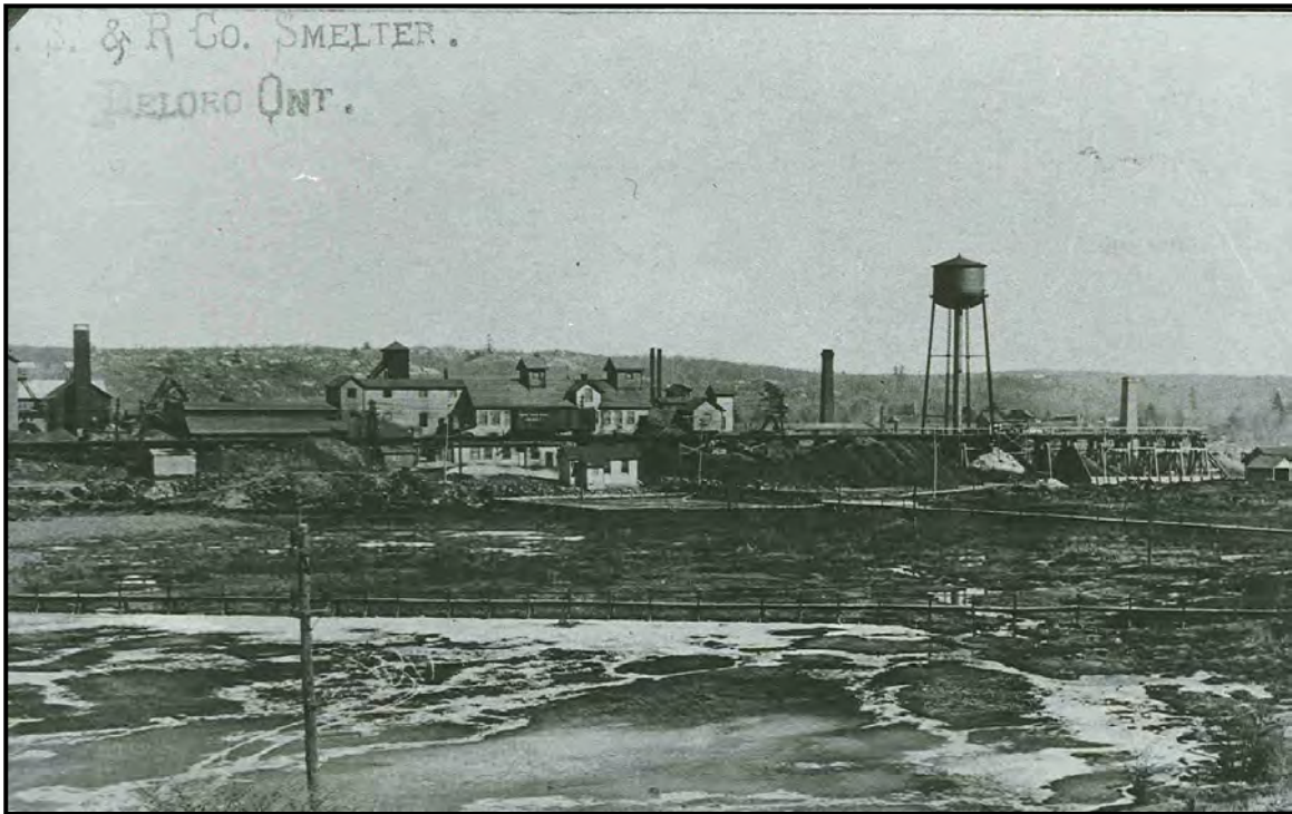
Plate 41: Industrial complex, c1920s showing boardwalk over wet land in foreground.
