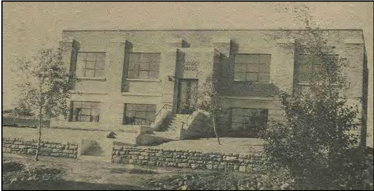
Plate 44: Newly constructed research laboratory, now the Arsenic Treatment Facility.
