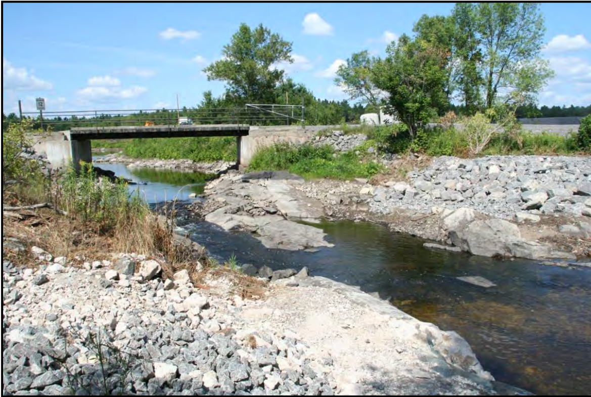
Plate 49: Following dam removal, August 2011. The bridge in background is in same approximate location as Plate 47
