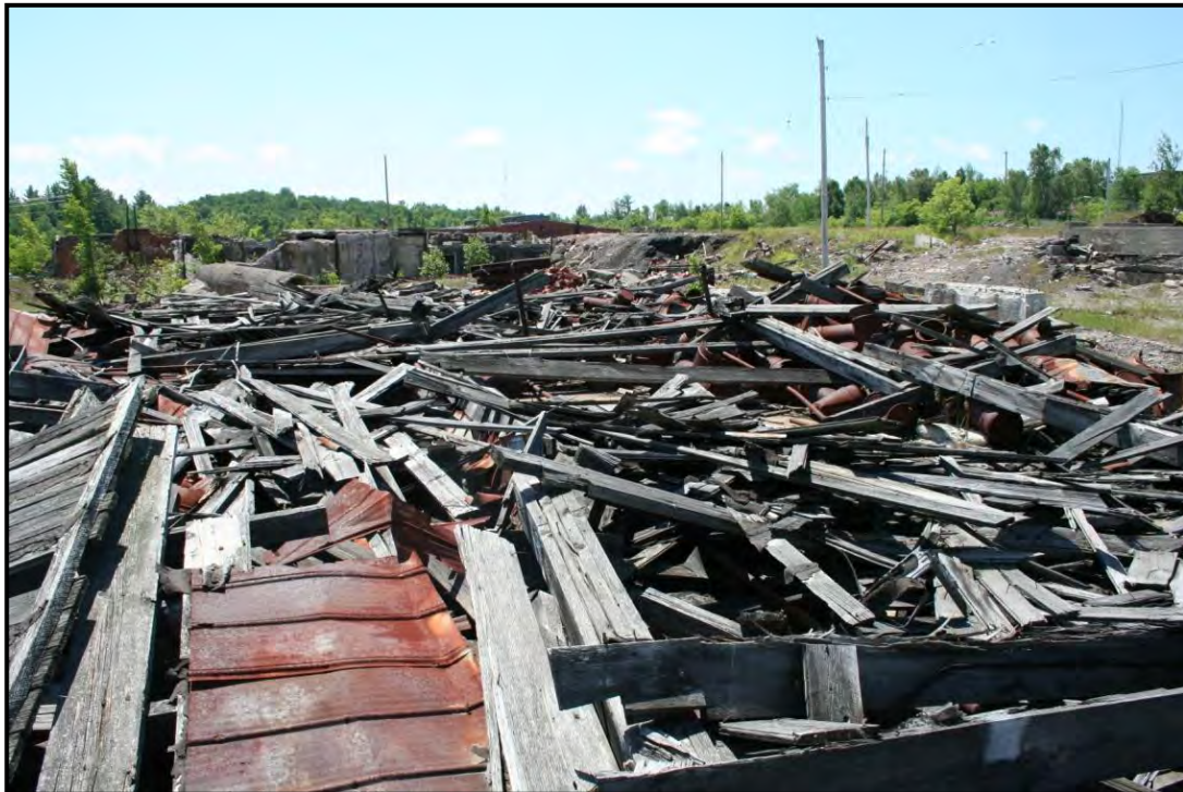
Plate 56: Cobalt oxide shed.
