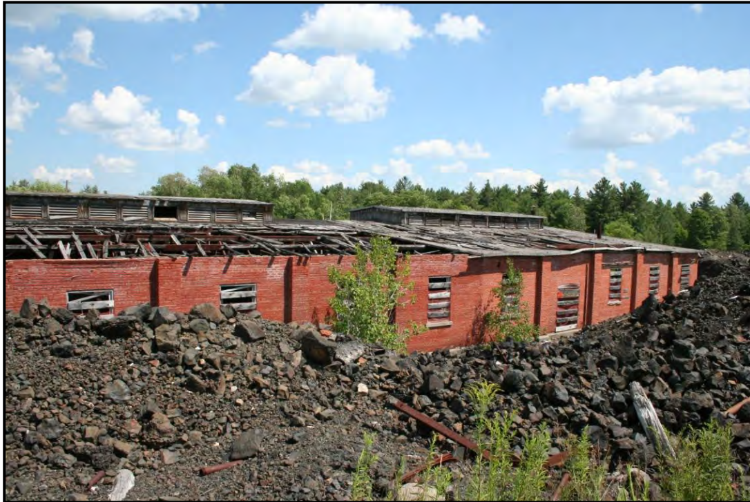
Plate 65: Slag pile beside Casting Building.
