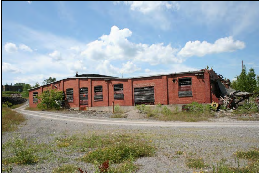
Plate 63: Exterior of Casting Building facing north.
