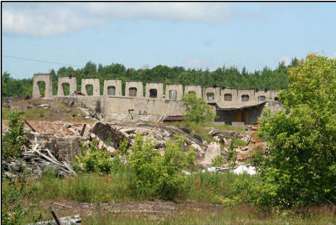
Plate 60: Primary Treatment Plant railway trestle.
