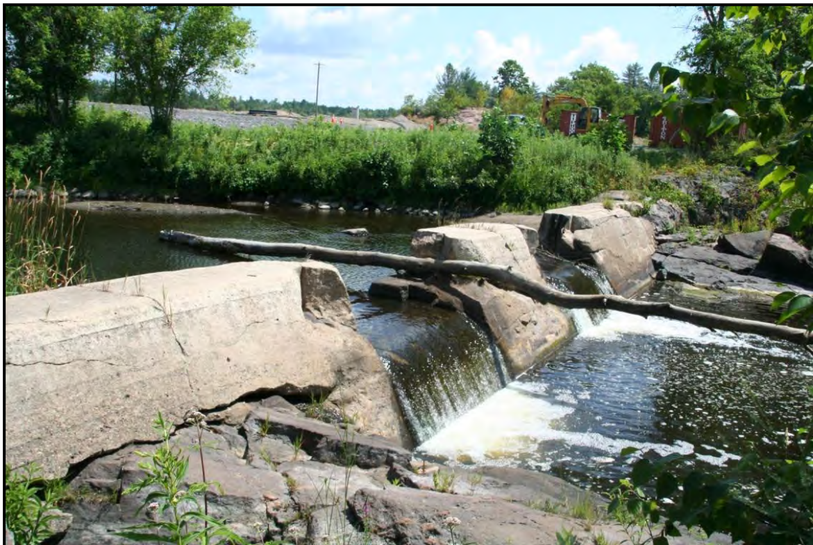
Plate 48: Dam across Moira River below road bridge in July 2011.
