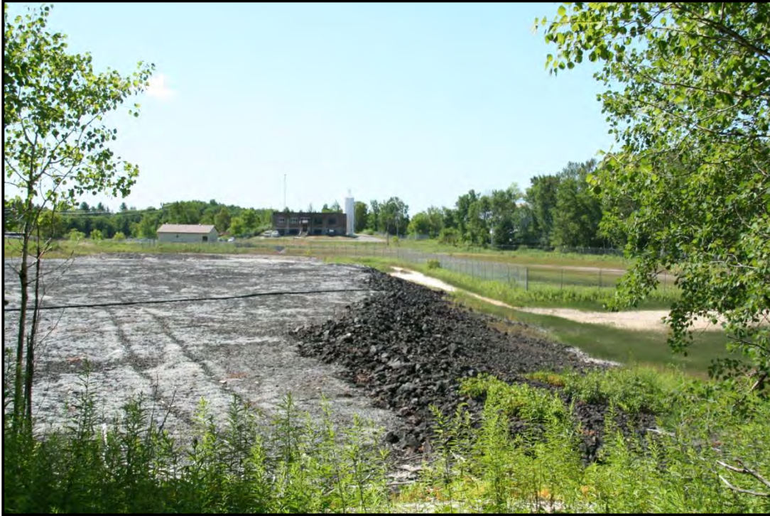
Plate 67: Calcium Arsenate Dump on left, fenced-in Equalization Pond on right and Arsenic Treatment Plant (former Research Lab) in rear..
