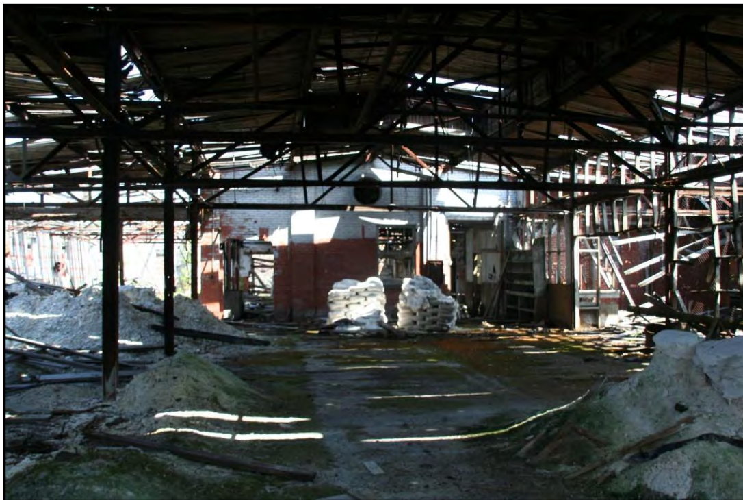
Plate 62: Casting Plant, interior.
