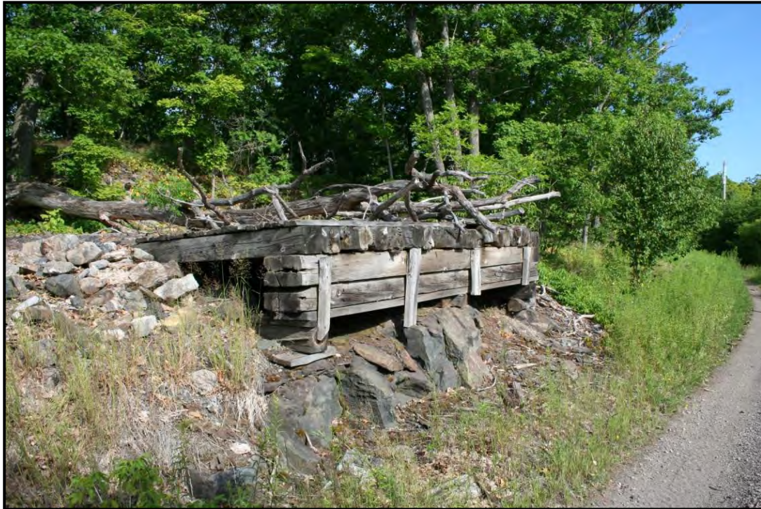
Plate 53: Initially identified as a “barber shop” but heavy timbers and layout close to former rail right-of-way suggest that this was a loading dock.
