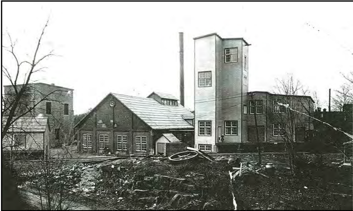
Plate 25: Air compressor and former generator in brick powerhouse in centre, transformer building on left, insecticide building on right, c. 1920
