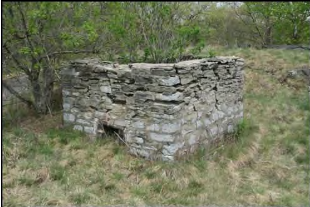
Plate 38: Powder Magazine with vent at base of shaft. See also Plate 27 for c.1900 view and Figure 11 for location
