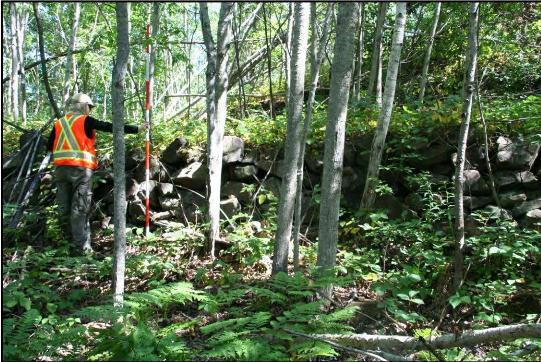
Plate 36: Stamp Mill Road showing stone retaining wall.
