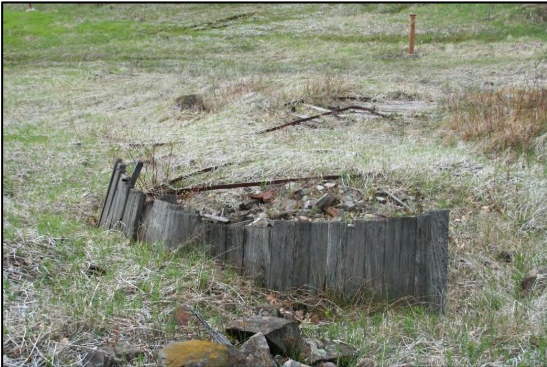
Plate 33: Wood tank adjacent to site of concentrator building.
