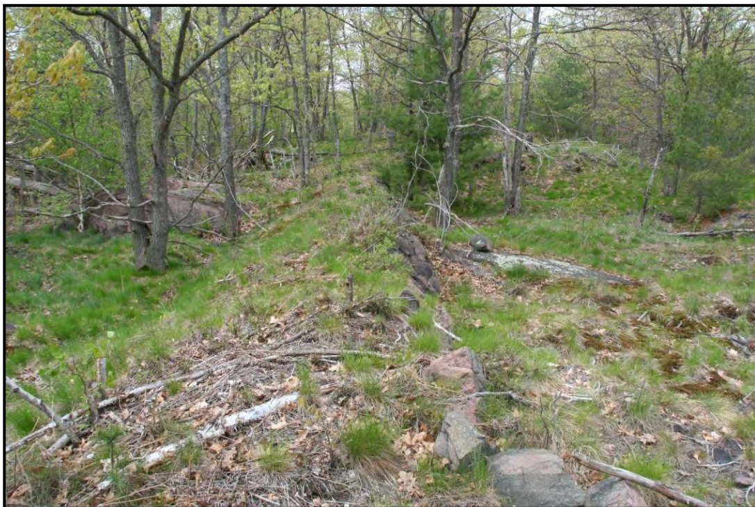
Plate 16: Dyke showing clay lining of dry stone wall to waterproof the structure. The head pond would have been in the valley on the left side.
