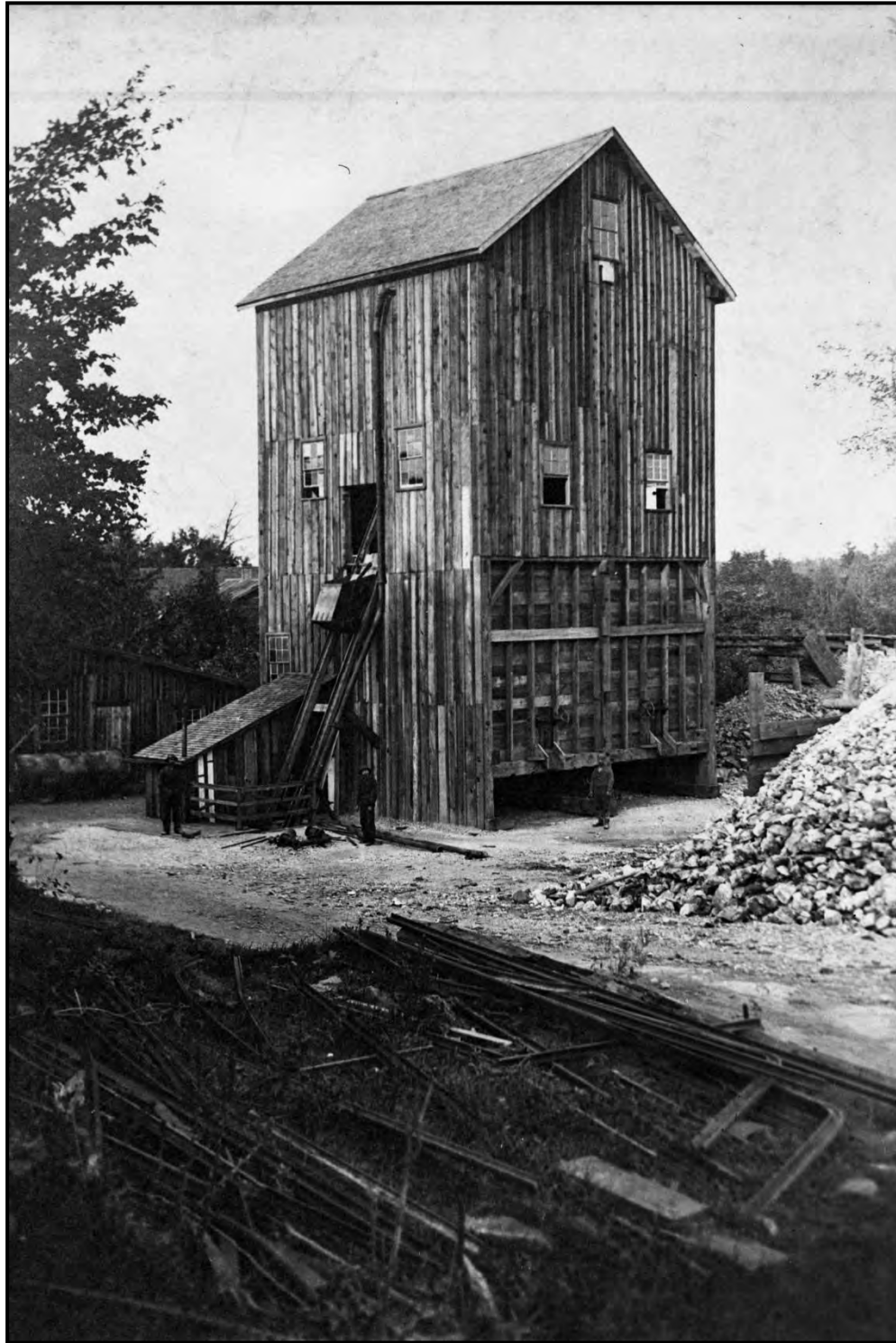
Plate 8: Gatling Shaft c.1900. A mine skip car is being hoisted into the hoist house and dumped into bins identified by the heavy timber framing on lower level of structure. Rock pile on right is low grade ore. Community Archives of Belleville and Hastings County, Deloro.
