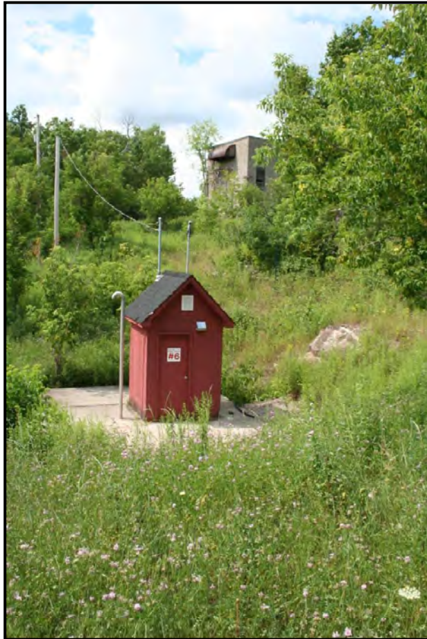
Plate 23: Modern Tuttle Mine pump house with 1907 electrical substation in background.
