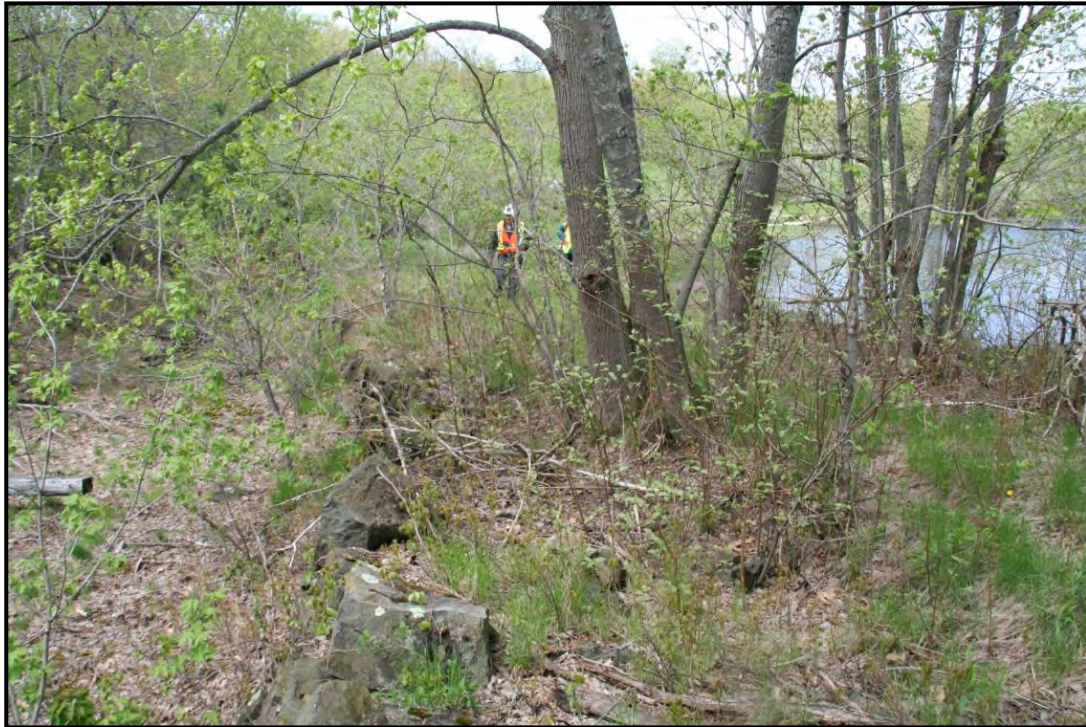
Plate 19: Top of tramway embankment with west wall visible on left; the east wall is between the two clumps of trees on the right.
