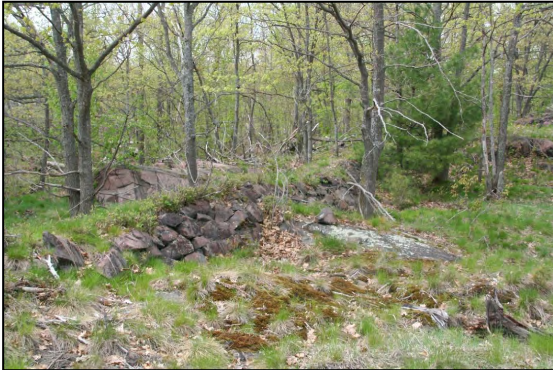
Plate 15: Dyke showing dry stone wall. The head pond would have been to the left of the wall.
