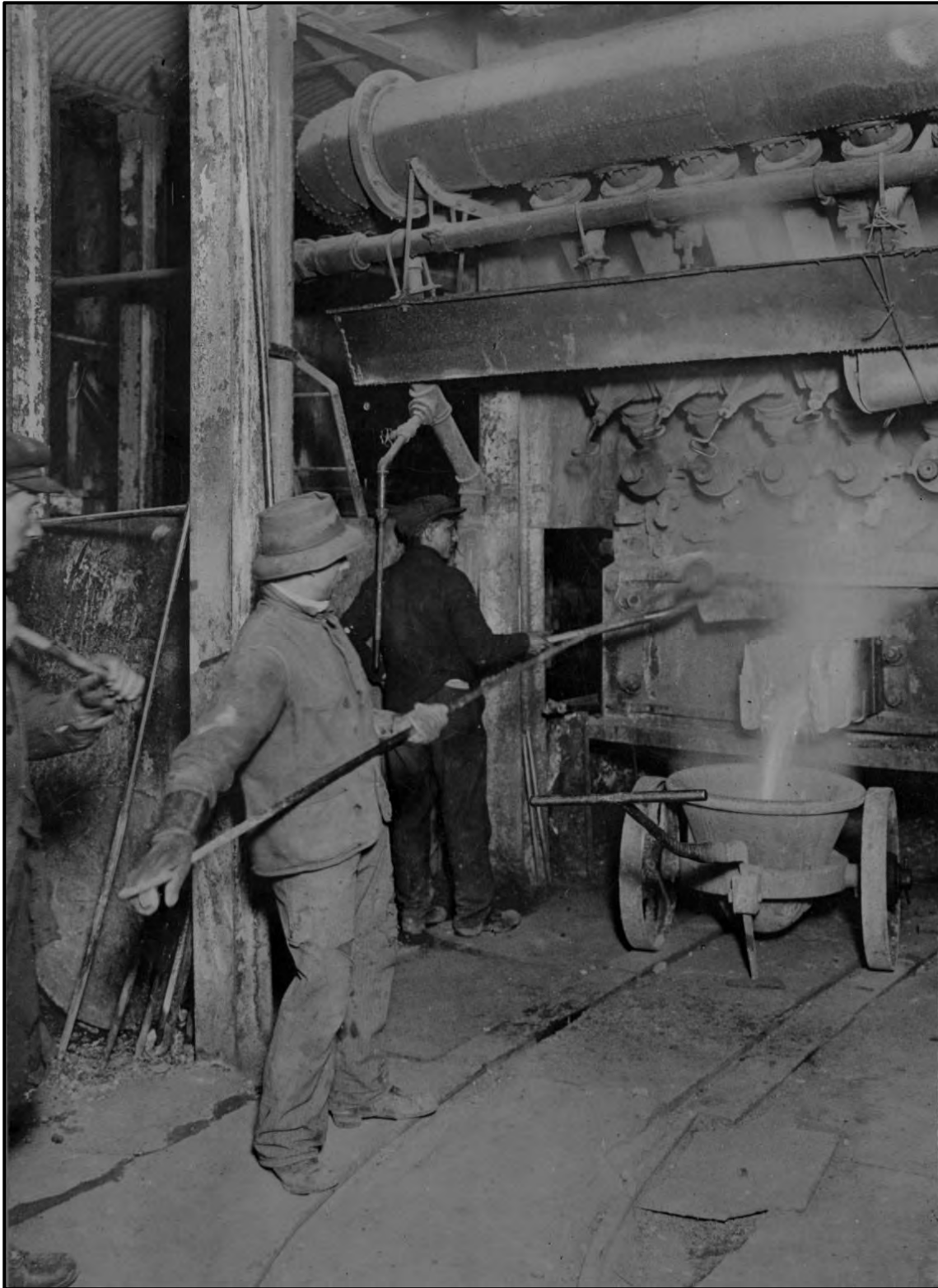
Plate 4: Tapping the blast furnace, Deloro 1908. Courtesy Deloro Stellite (C. R. Wittemore)/67. Negative by Lumbers.
