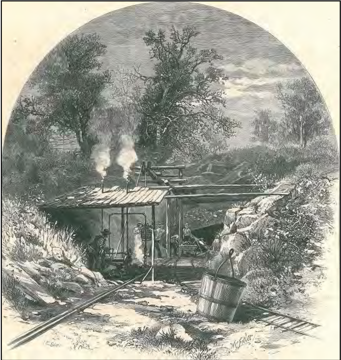
Plate 3: Iron mining at Marmora c.1880 illustrating an adit. Steam engine hoist over mine shaft; two iron pipes on left for compressed air or steam for drills, tramway track on right with bucket for ore. Picturesque Canada
