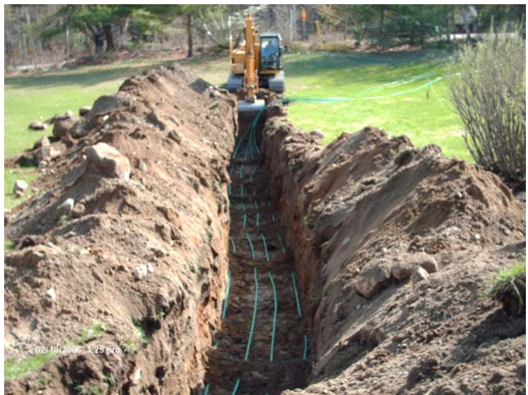
Figure 6: Photograph of Horizontal Closed Loop Partially installed 7
