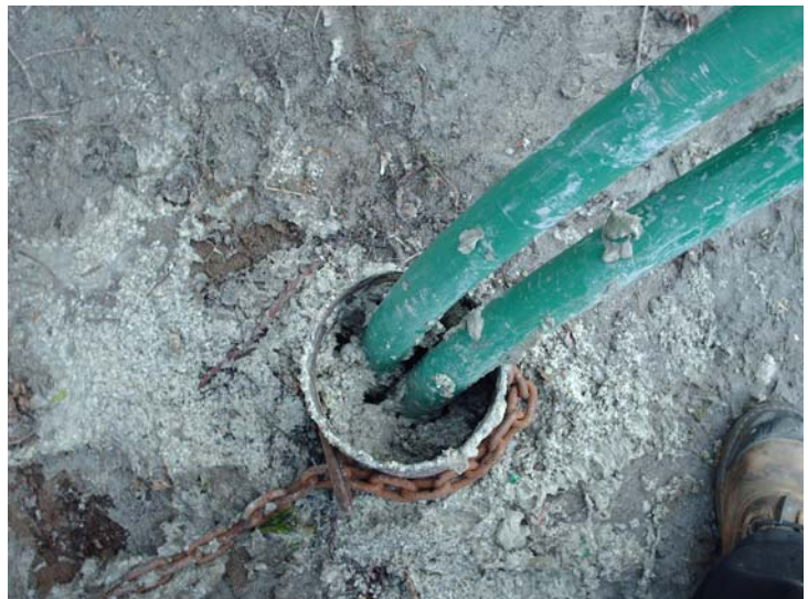
Figure 4: PHOTOGRAPH OF A CLOSED VERTICAL LOOP INSTALLED IN A VERTICAL BOREHOLE 5
