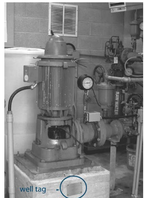
FIGURE 13-20: WELL TAG ON EQUIPMENT ASSOCIATED WITH THE WELL AS CLOSE AS POSSIBLE TO THE CASING
