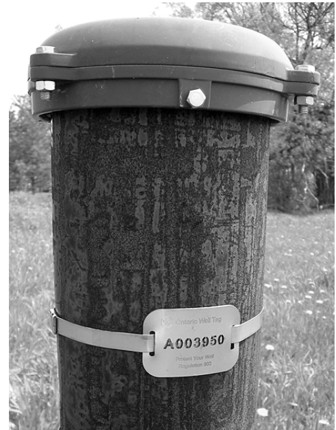
FIGURE 13-17: EXAMPLE OF PROPERLY ATTACHED WELL TAG
