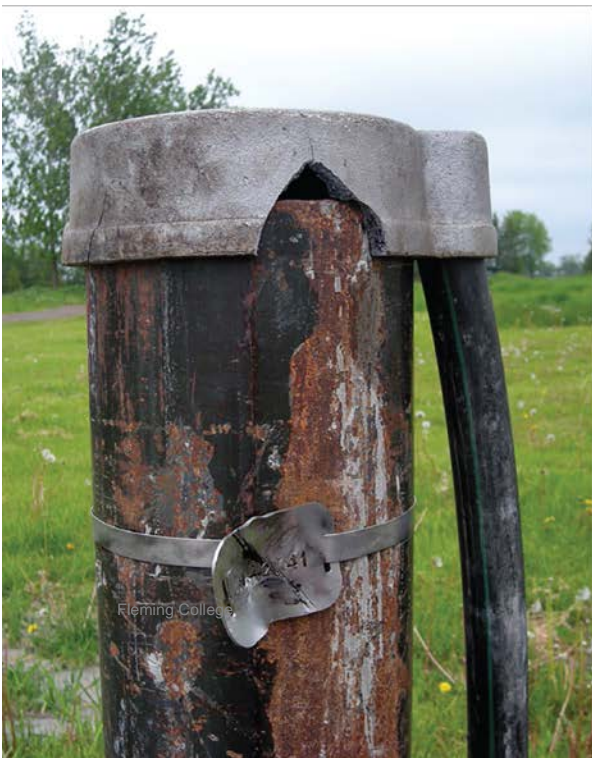
FIGURE 13-22: BEFORE - WELL TAG MUST BE REPLACED
