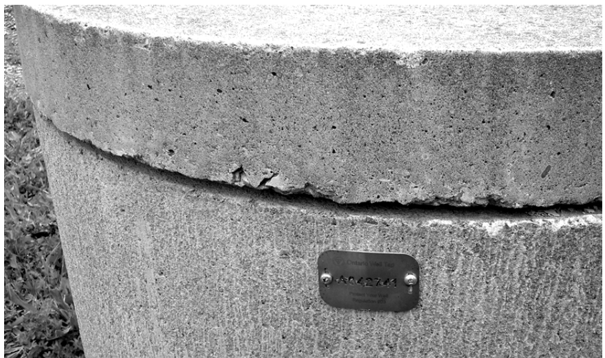
FIGURE 13-18: THREADED SCREWS ATTACHING WELL TAG TO CONCRETE CASING
