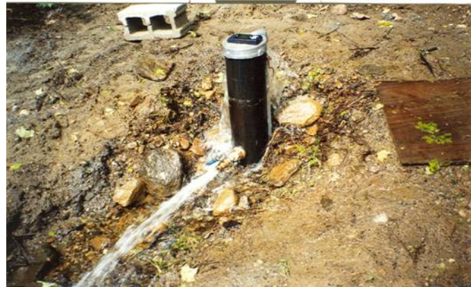
FIGURE 12-16: UNAPPROVED BURIED FLOW DISCHARGE PIPING WITH SUBMERGED INLET 8
