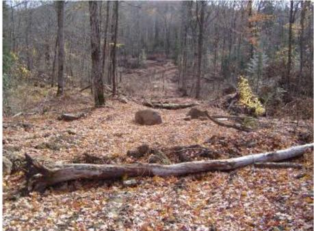
Figure 5.2f. Rehabilitating main skid trails by stabilizing crossings [top], installing water bars on slopes [bottom], and other means can reduce the risk of future erosion (photos by Bancroft Minden Forest Company Inc.).
