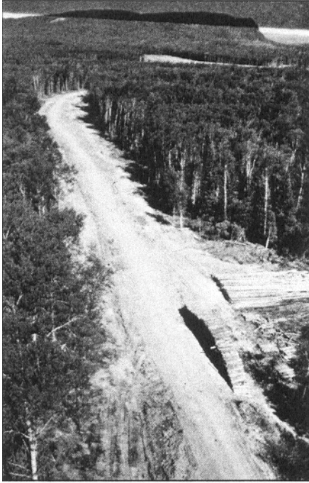
Timber cut from the right-of-way clearing should be utilized.
