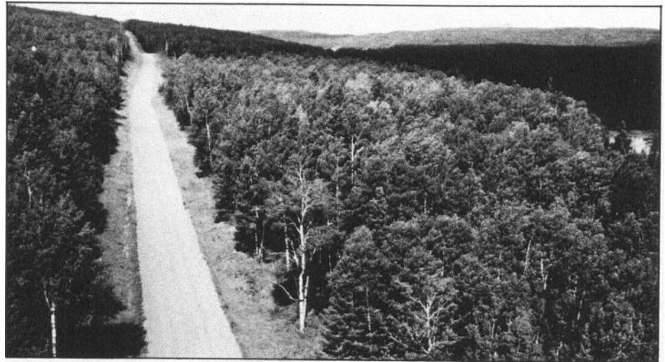
Good aesthetics on this road are created with a straight alignment, push-outs and good re-vegetation.
