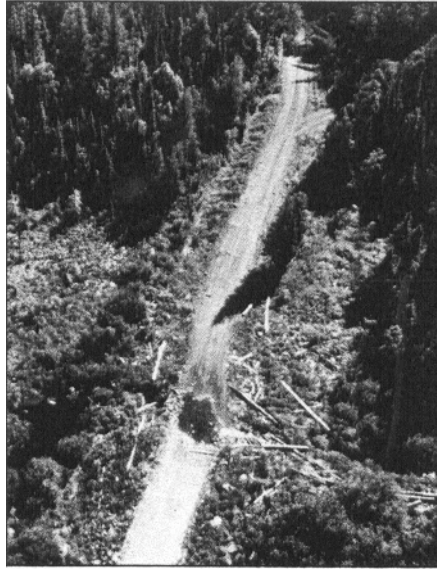
Failure to maintain culverts and ditches may lead to a road washout.
