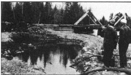
A cofferdam allows abutment construction in an area isolated from flowing water.
