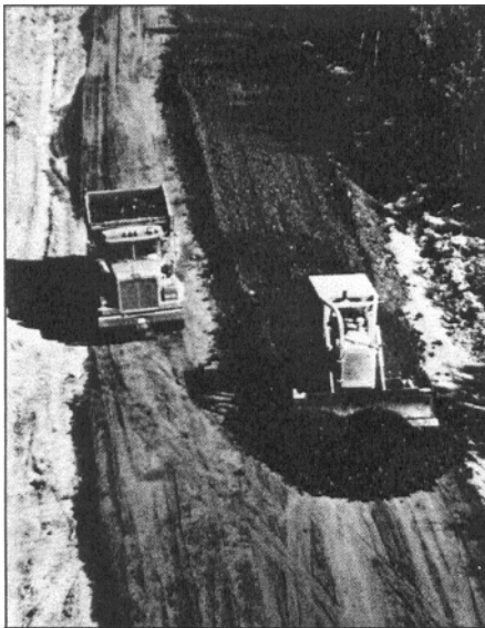
Fill construction in shallow, full-width layers ensures a stable road bed.
