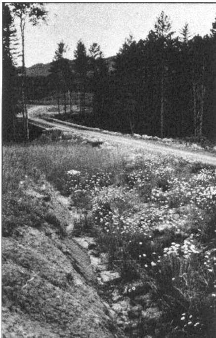
Re-vegetation around a water crossing will help to filter sediment.
