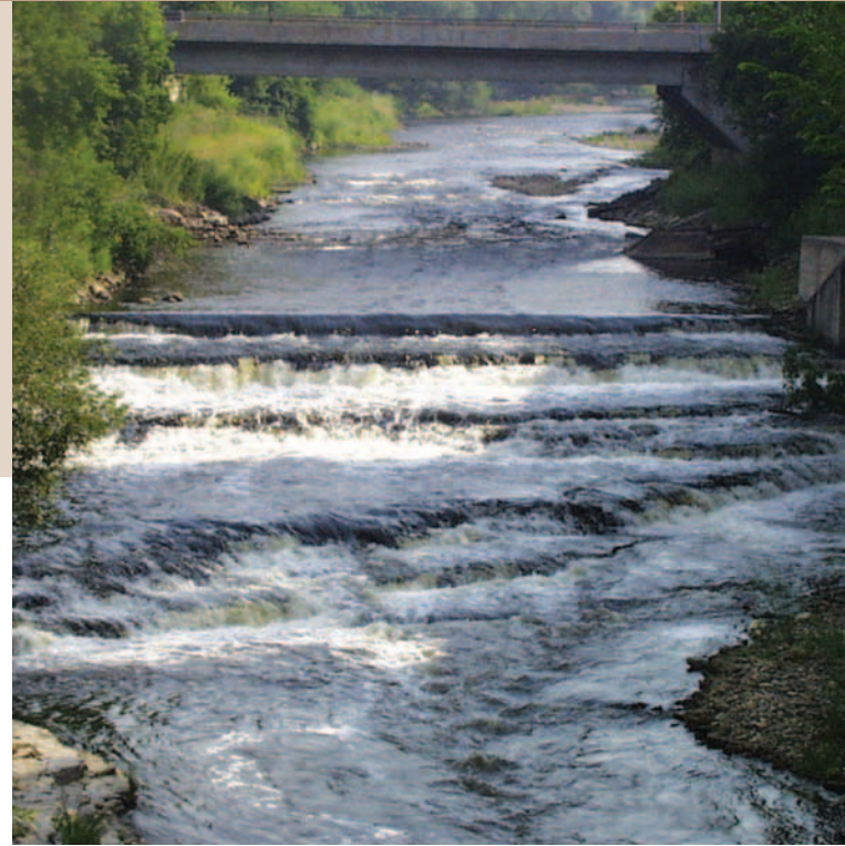
Beatty Dam, Grand River – After dam removal
