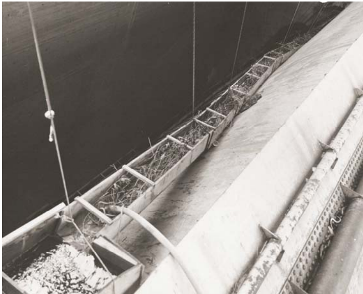
Figure 23. Top span of the prototype wooden eel ladder at the Moses-Saunders hydroelectric station on the St. Lawrence River. Photo shows willow cuttings in the ladder with a resting pool (bottom left) (Ontario Ministry of Natural Resources photo).
